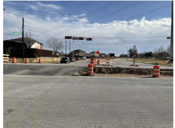
Hickory Creek, West of Teasley Lane — Looking East
