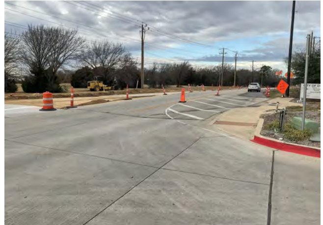
Hickory Creek Road — Sprout's West Driveway, Looking Right
