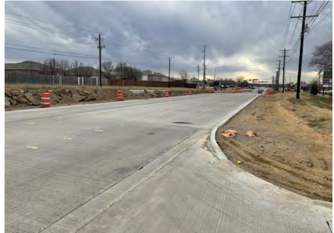
Teasley Lane — Northern Sprouts Driveway, Looking Right
