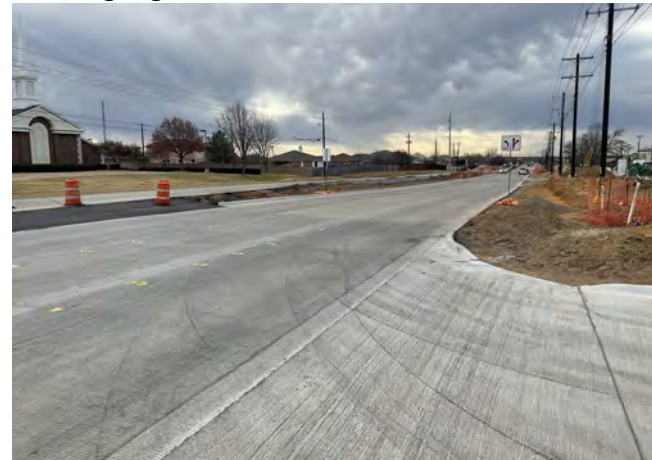
Teasley Lane — Existing Driveway 1, Looking Right
