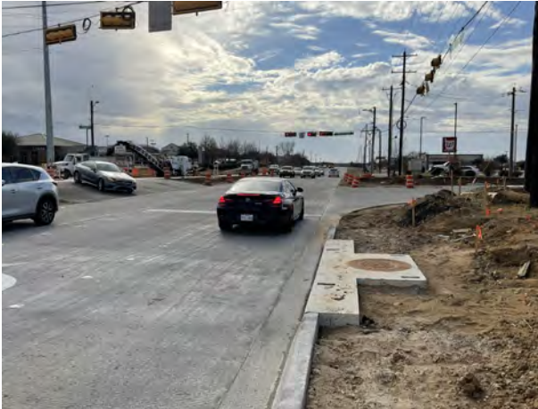
Teasley Lane, North of Hickory Creek Road — Looking South
