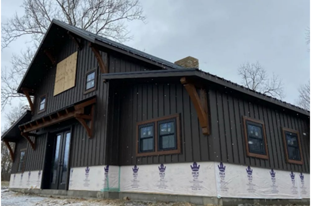
Example of prefinished aluminum batten board
